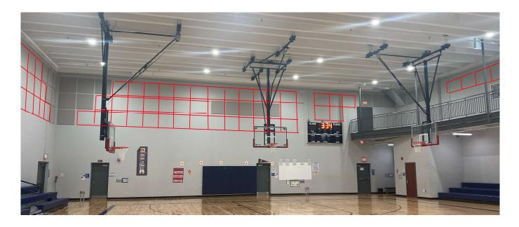
**4'x8' Layout** would leave the existing panels in the corner, but remove middle panels. 4'8 panels would be added evenly around the space
